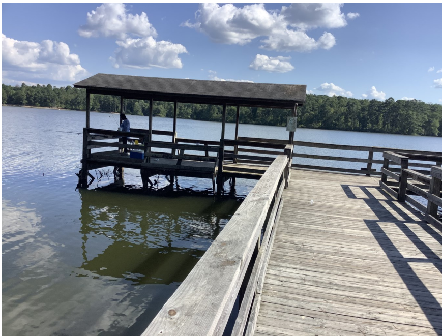
Figure 1. Fall is a good time for pier construction or maintenance.
