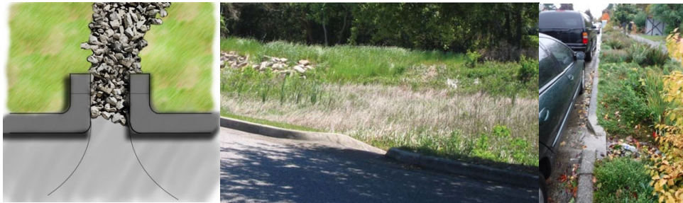
Figure 78: Curb cuts allow water to flow into a vegetated area.
