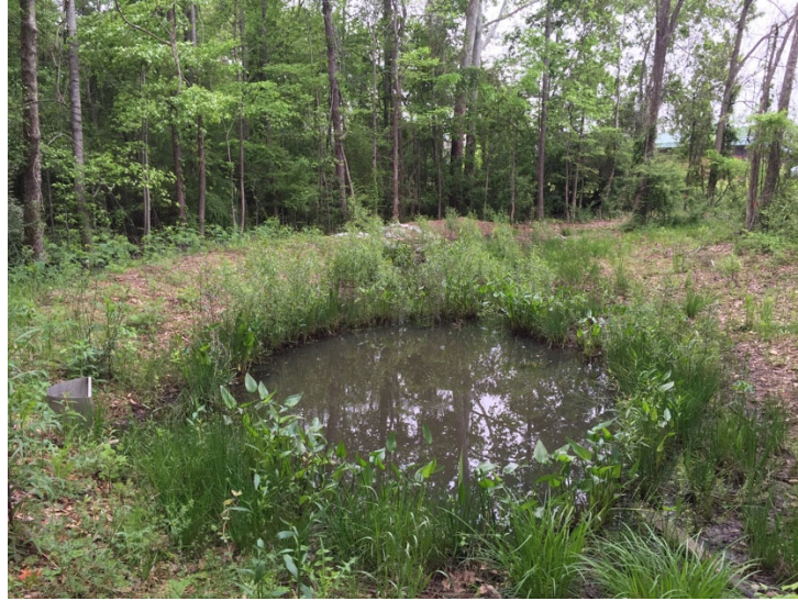
Figure 72: Constructed stormwater wetland.
