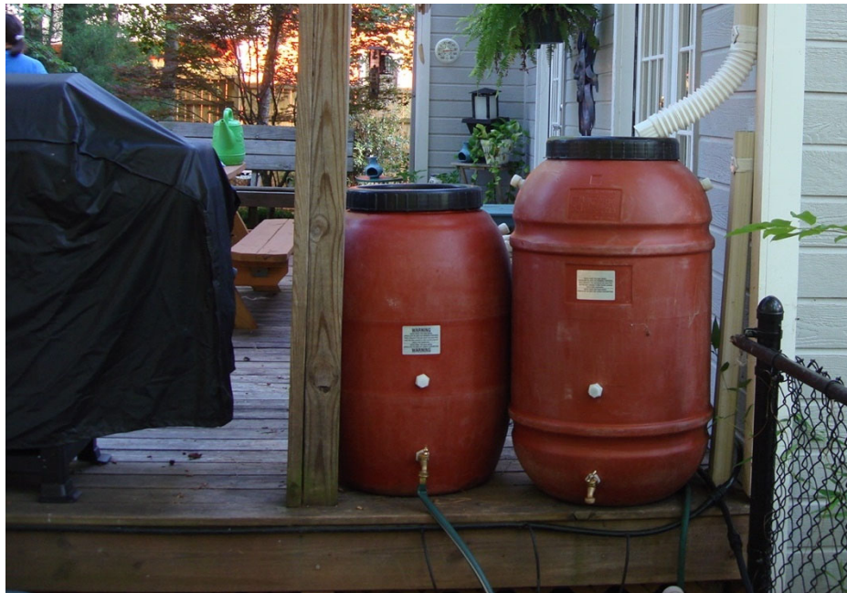
Figure 75: Rain barrels in a residence, connected to garden.
