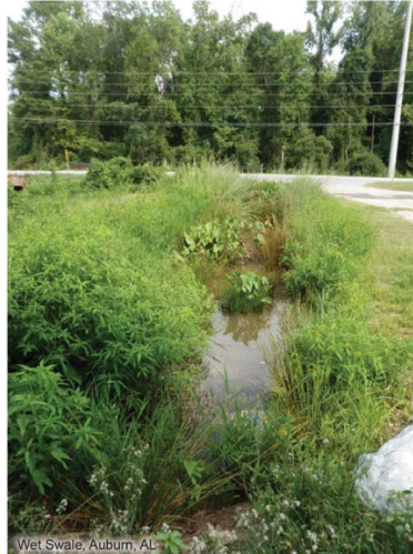
Figure 74: Wet swale along a roadway in Auburn, AL.
