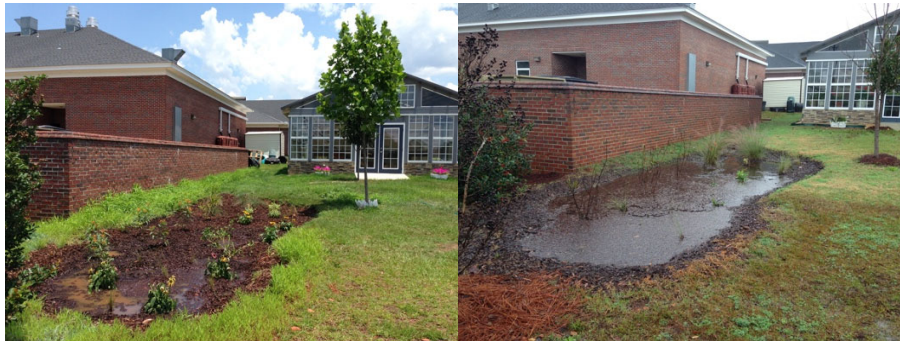
Figure 76: A newly planted rain garden begins to serve its function.
