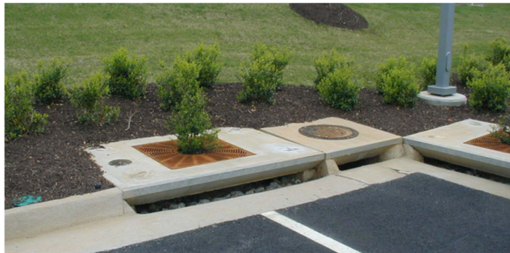
Figure 80: Newly installed Filterra Tree Box. Source Contech Engineered Solutions.
